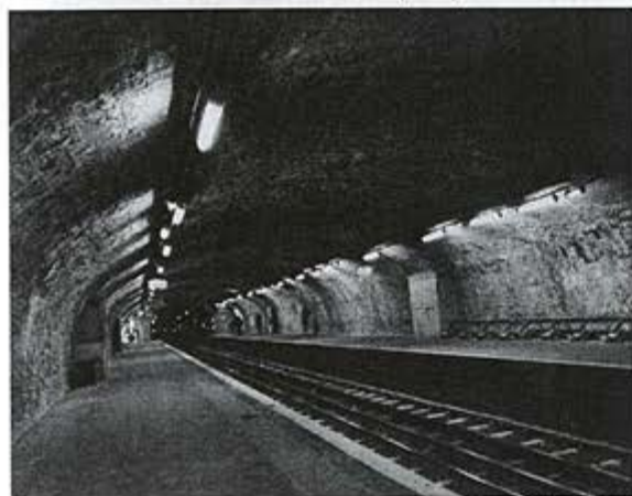
© RATP - SUTTON Denis 209289 - 22/02/1993 Modernisation de la station Buzenval (1993)
