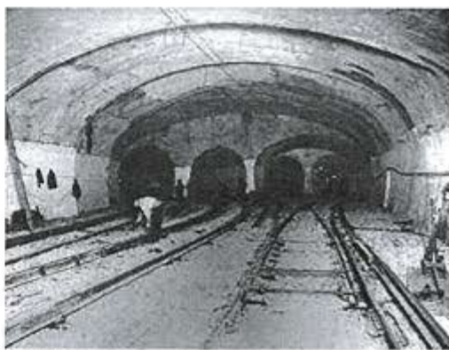
© RATP - ND 4281 - 07017 Construction de la station Gambetta (1905)
